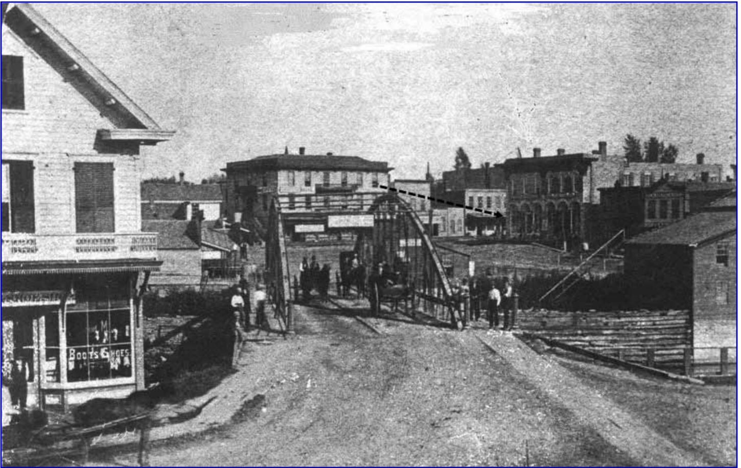
West side view of the steel bridge in the foreground crosses the Cannon River and leads toward Mill Square. A black arrow from the three-story structure, Dampier House Hotel, denotes Wheeler’s position of fire from the 3 rd floor of the hotel. (Photo Courtesy of Hayes Scriven, Executive Director of Northfield Historical Society, Northfield, Minnesota.)
